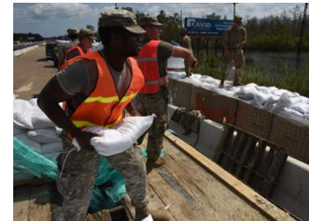
South Carolina National Guard Engineers and Transportation Soldiers place sandbags along the road to prevent flooding in the aftermath of Hurricane Florence, Sept. 2018. By Senior Master Sgt. Edward Snyder
