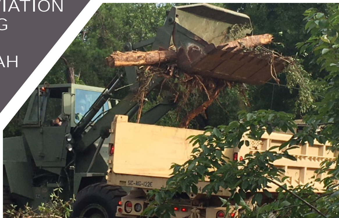
The South Carolina National Guard engineers conducted their annual training at the Savannah River Site, June 2018, performing construction on the parking lot. Courtesy photo
